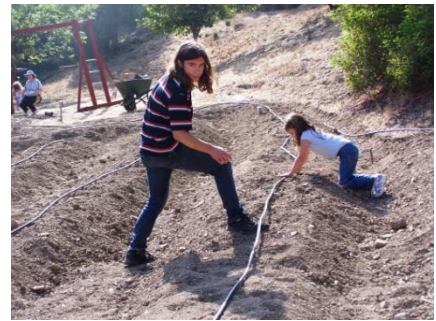
Christopher and Katherine laying and stapling the tubing
