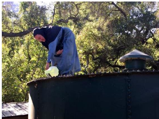
Pouring chlorine into the water tank – last time
