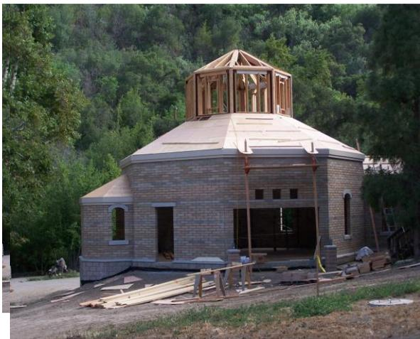
As can be seen from the photo to the left, the new chapel is turning out to be very, very beautiful. At this stage, the outer walls are finished and the roof is partly in place, so that the outward form of the building is apparent. Much remains to be done, of course, before the chapel is completed and can be used. *The immediate need is to install the windows and doors* so that the building can be enclosed. However, at this time, we have only a portion of the funds needed for this
